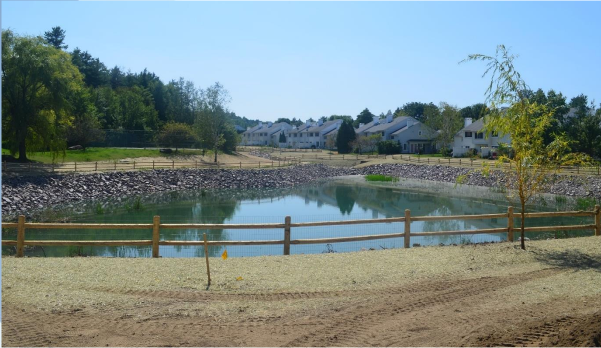
View of Village at Dorset Park Pond 3 – Project included the upgrade of 3 stormwater treatment ponds to current standards.
