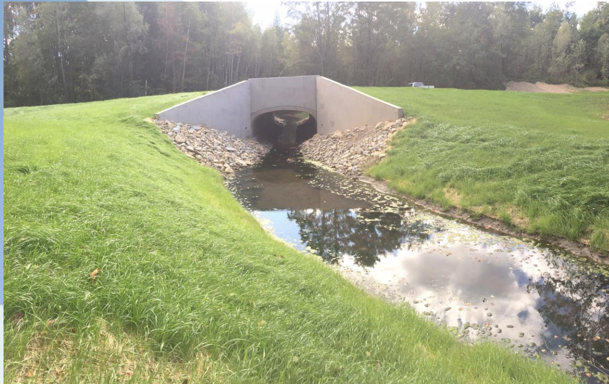
View of Replaced Culvert Facing Upstream
