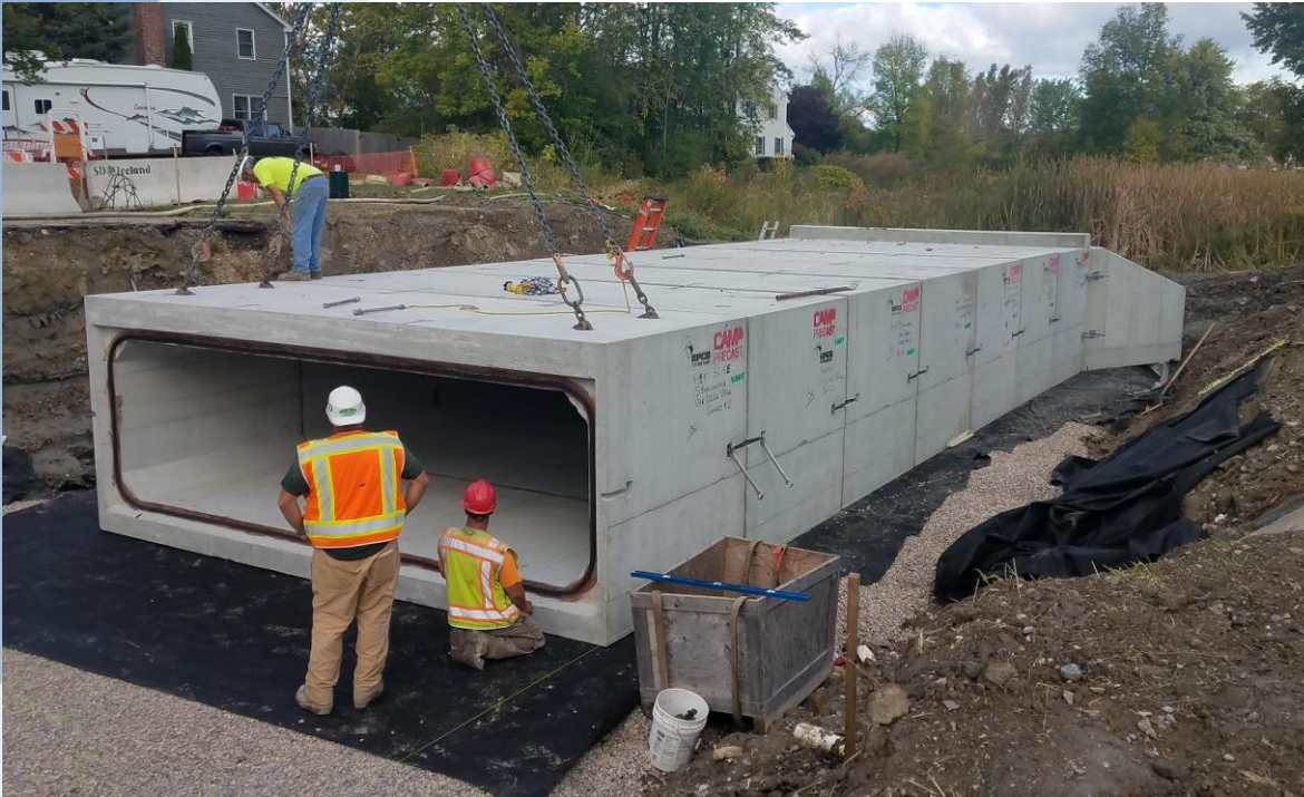
Placing Precast Culvert Sections Under Moss Glen Lane – The project included replacement of two undersized culverts in Oak Creek Village
